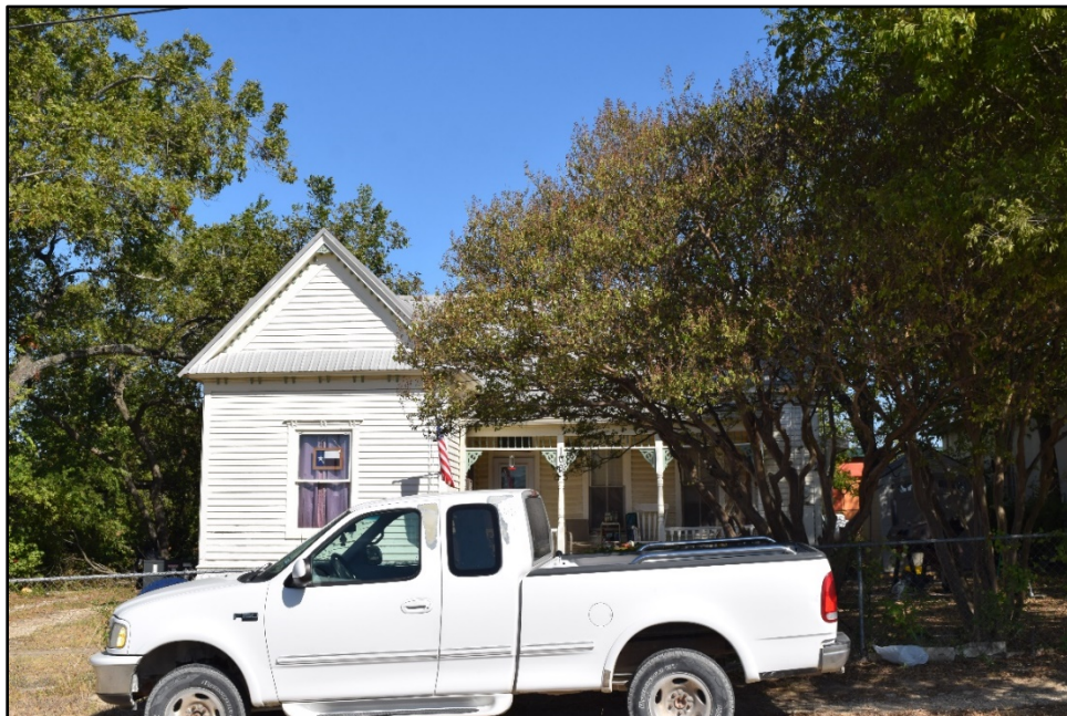
Figure 17. Historic-age residence immediately north of project area, south (front) elevation, facing north.
