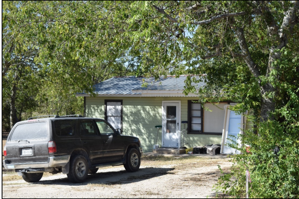
Figure 18. Historic-age residence immediately south of project area, east (front) elevation, facing southwest.
